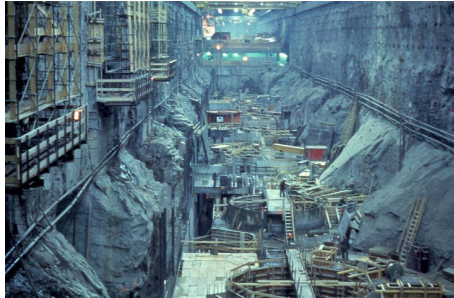
The LG2 James Bay station, under construction in 1978
